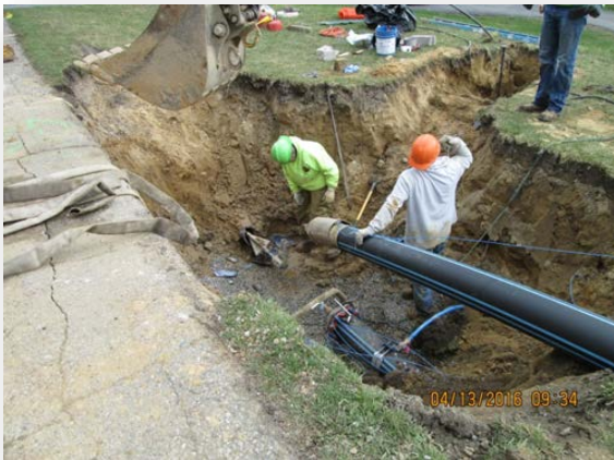
Bursting head and HDPE pipe at entrance pit
