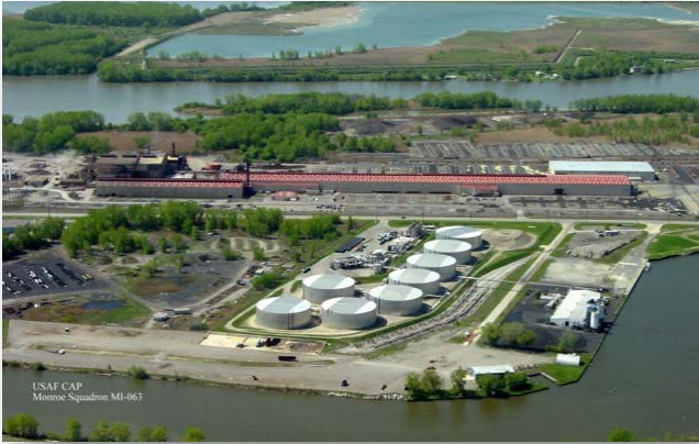
Aerial view of future dredging operations
