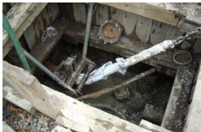
CPP liner being stretched
