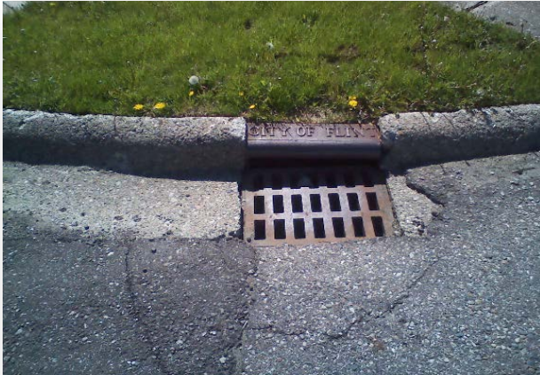
City storm sewer catch basin
