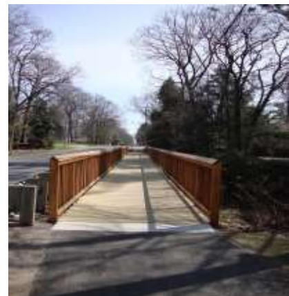
Elevated Wooden Walkway (138.5' L x 8' W)
