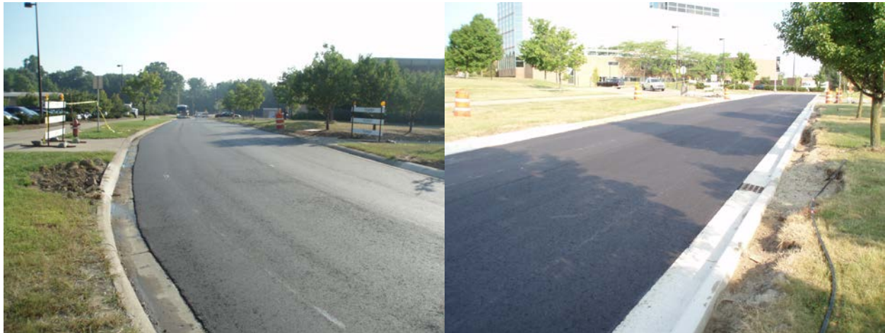
Completed and Open to Traffic
