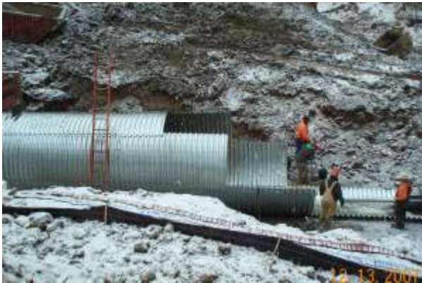
Plate Pipe Replacement
