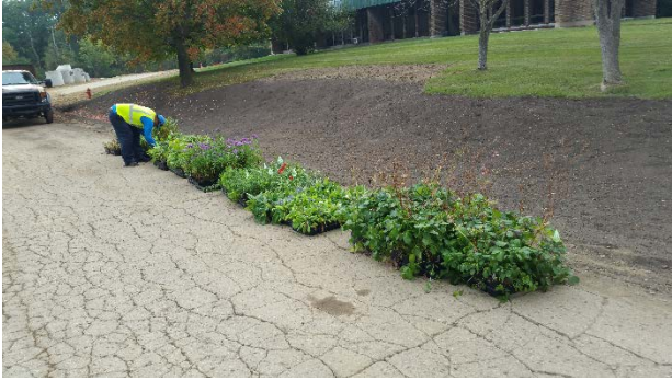
Vegetated Swale Plant Installation
