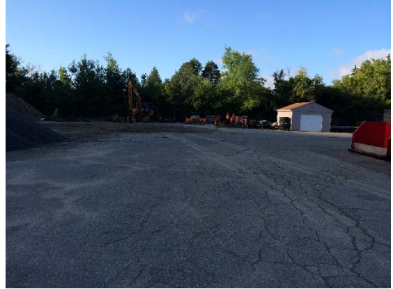
Existing Asphalt Parking Lot & Materials Storage Area
