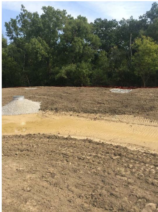
Detention Basin Installation
