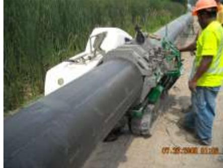
**HDPE Pipe in Fusion Welding Machine**
